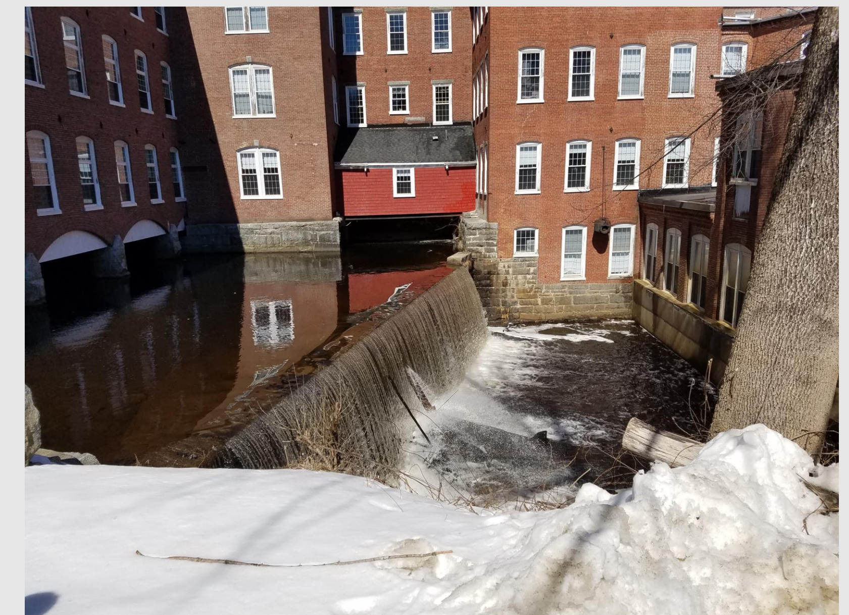
The Lower Dam at Sawyer Mill Apartments in Dover, NH. Dam to be removed in summer 2018.
