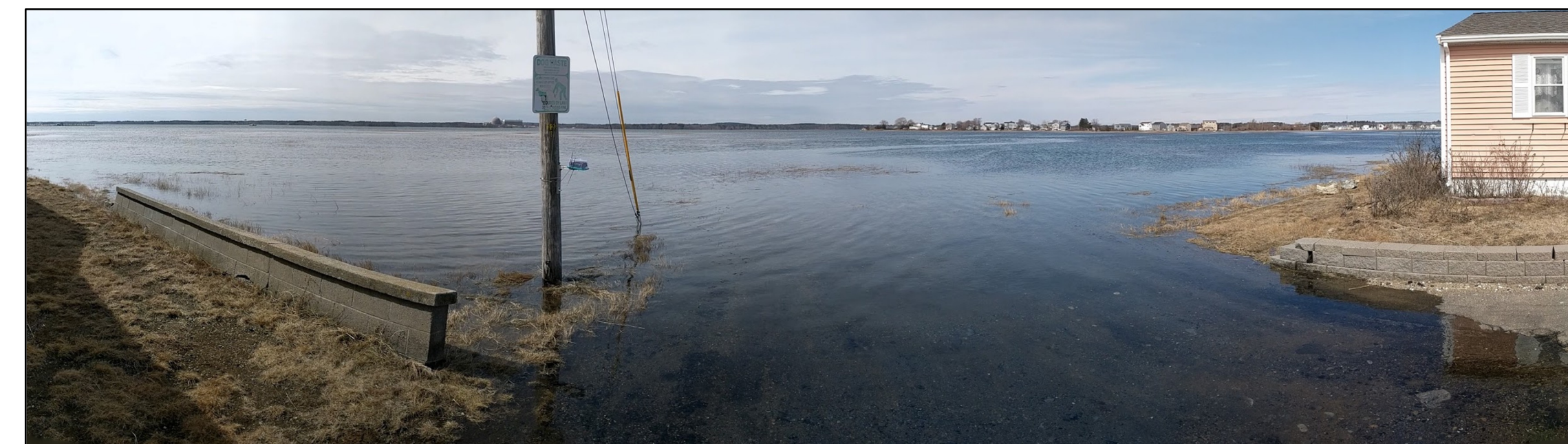
Figure 5: A small ultrasonic sensor (center left, on the telephone pole) records the water elevation as it floods onto Hobson Ave.
