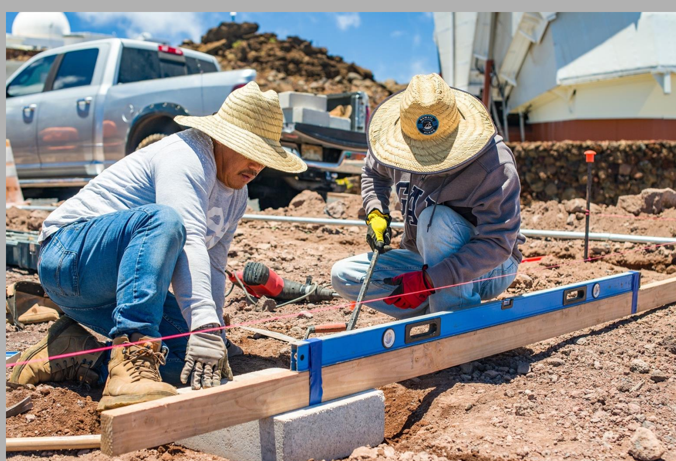
Figure 3. Work being done to prepare the site on the summit of Haleakalā
